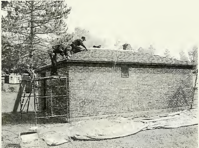
New Roof Installation at JImtown CL2 Station
